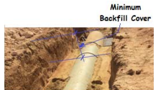
Minimum Backfill Cover
